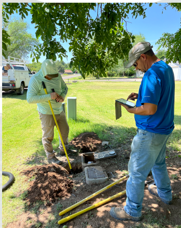
Fig. 1: Staff digging up and visually inspecting water lines for material verification and classification.
